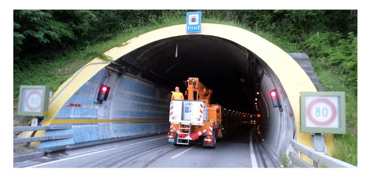
The project concerns inspections in the years 2013, 2018 and 2023 for tunnel Schweizerhalle (1030 m) and tunnel Arisdorf (1349 m). After a first KUBA training phase, the structures data have been defined and collected; the main inspection (control, analysis and evaluation of each single structural element) and, finally, the final documentation with the proposed intervention concept have been performed.
